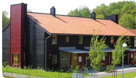
20 terrace houses using passive house technology have been built in Lindås. They have no conventional active heating systems, with most of the heating being provided passively from the occupants' body heat, by surplus energy from various domestic appliances and by insolation.
